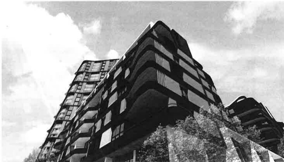
Street Level View_Corner of Hill Road & Burroway Road
